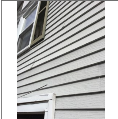
Repair area above garage door
