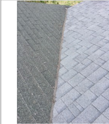
Two different shingles
