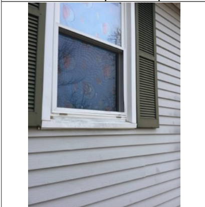
Broken storm window. Old wood window needs repair or replaced
