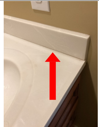
Suggest ceiling vanity top to splash as a preventative measure
