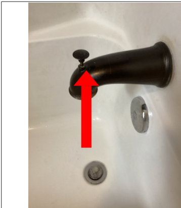
Tub diverter is stuck
