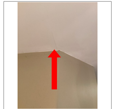
Typical cracks along drywall seams
