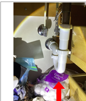
Slowly dripping underneath the drain line of the left sink
